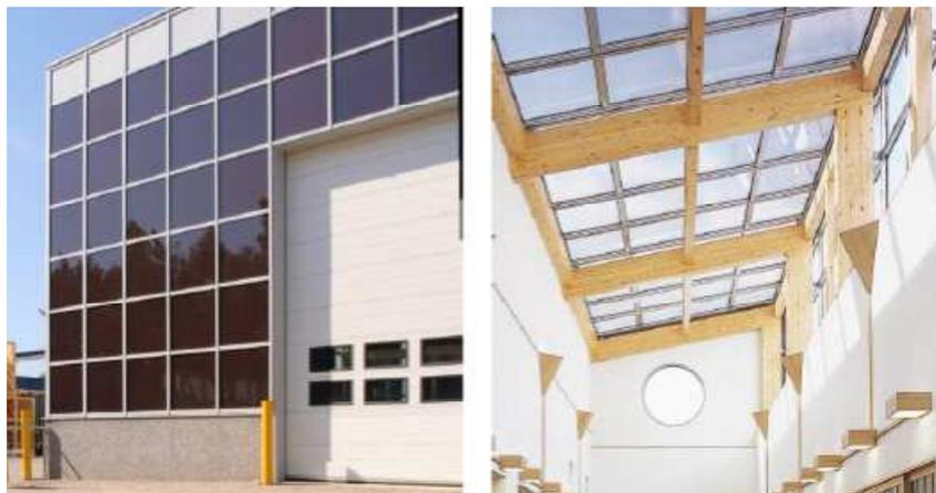
Figure 6.3.1: Examples of integration of modules in façade and canopy
