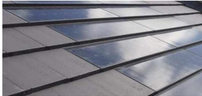
Figure 3.3: Overall Picture of a roof with Solar Century tiles
