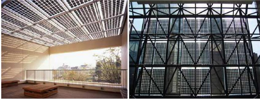
Figure 6.2.1: Example of integration of translucent modules
