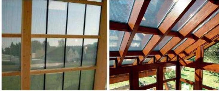
Figure 6.3.2: Example of façade integration and canopy of semi-transparent panels Schott-Solar
