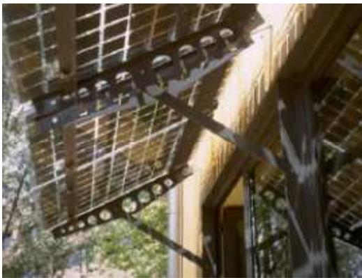
Figure 6.1.2: Fixing of the modules by boring in zones without cell
