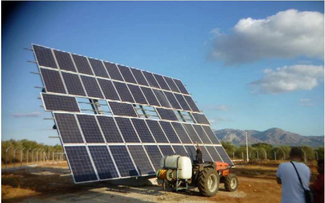
**Figure 3 - Cleaning of a small-scale PV installation by jetting water.**
