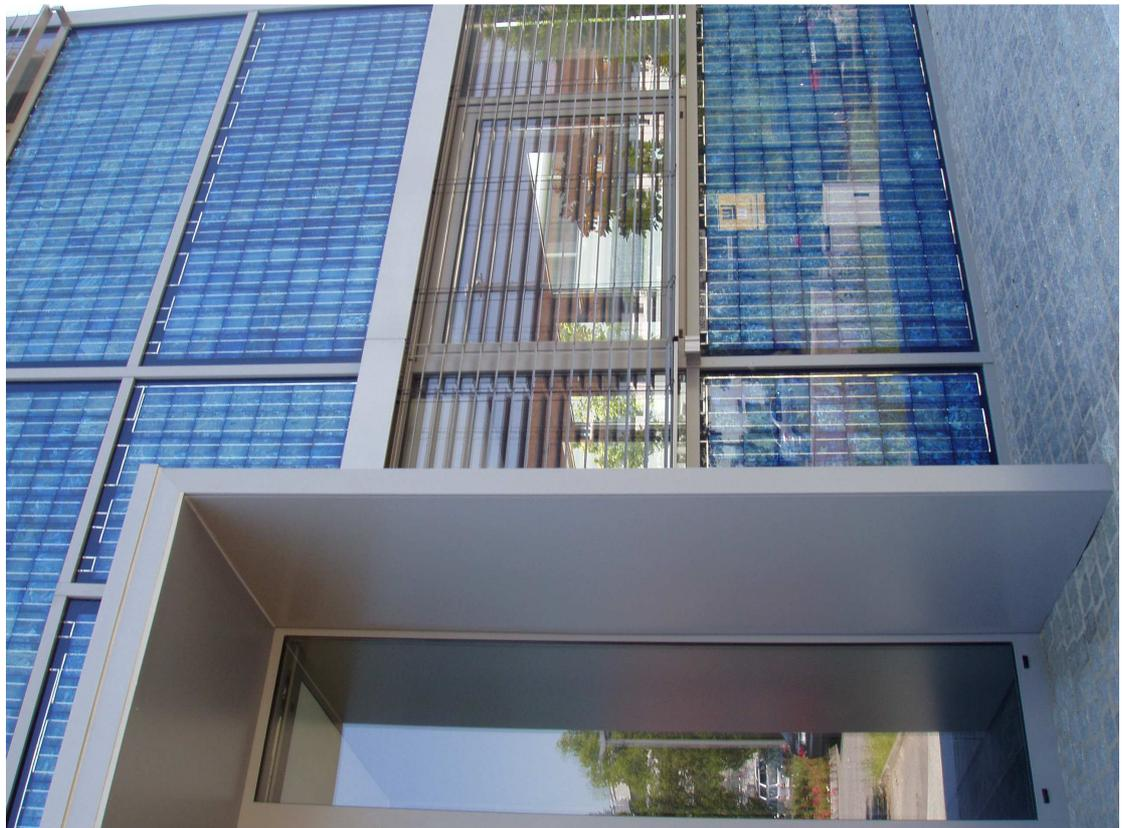
**Figure 5 - Polycrystalline PV panels retrofitted to cover the facade of a commercial building. They were used to replace mirrors.**
