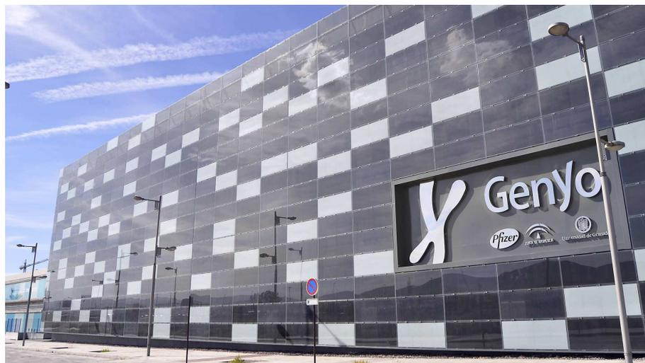
**Figure 4 - Pfizer-University of Granada-Junta de Andalucía Center for Genomic and Oncologic Research (GENyO) ventilated photovoltaic façade designed by Onyx Solar. It generates about 32 MWh/annum.**
