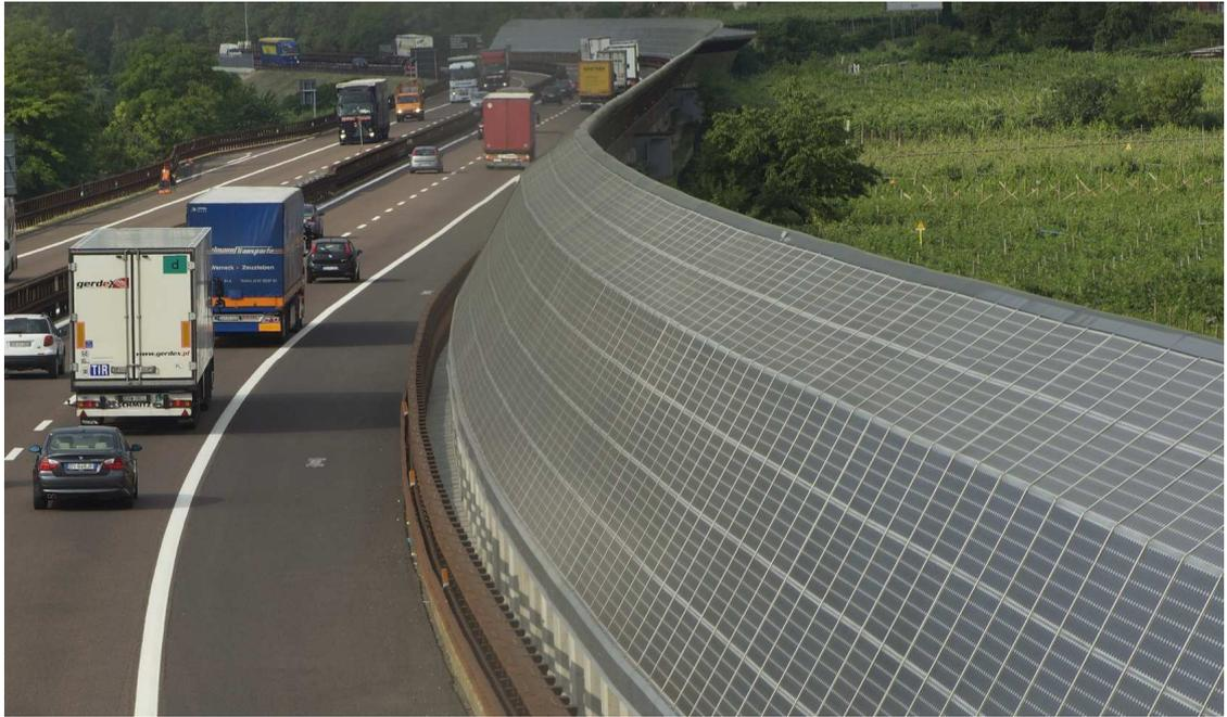
**Figure 2 - Medium-scale PV installation acting as a highway sound barrier. Brenner Motorway, outside the town of Marano, Italy.**
